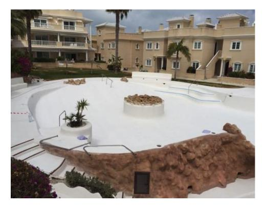
Pool, calcium mortars treated with CONTROLL®INNERSEAL and CONTROLL®TOPSEAL
