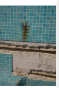
✓ Sealing joints, filling with mortar and nanocristalization in areas open for tastings.
