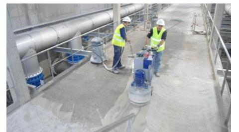
ROUGHING AND NON-SLIP FINISH + CONSOLIDATION AND RESISTANCE TO ABRASION WITH NANOCRISTALLIZATION
